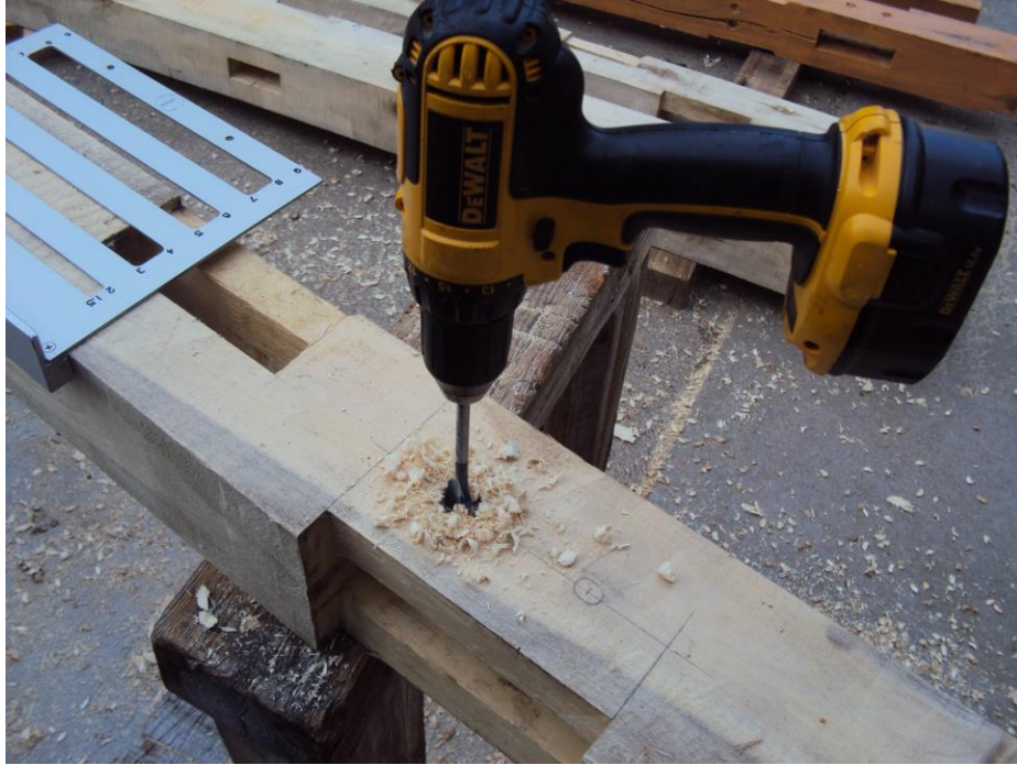
Drilling a Peg Hole
