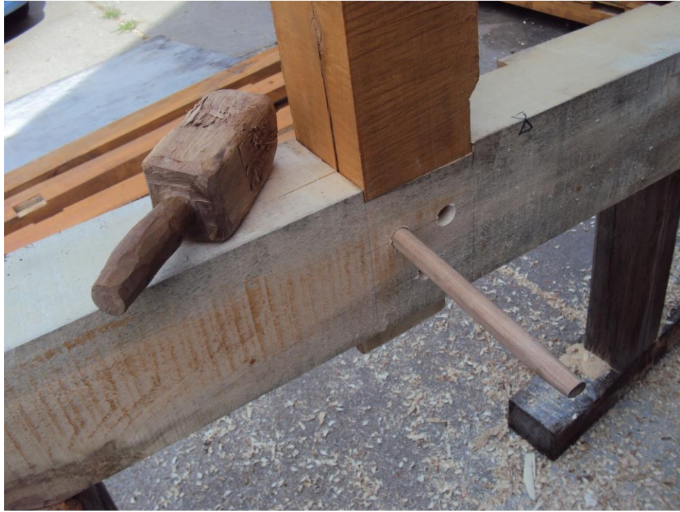
Test Fitting & Marking Peg Hole
