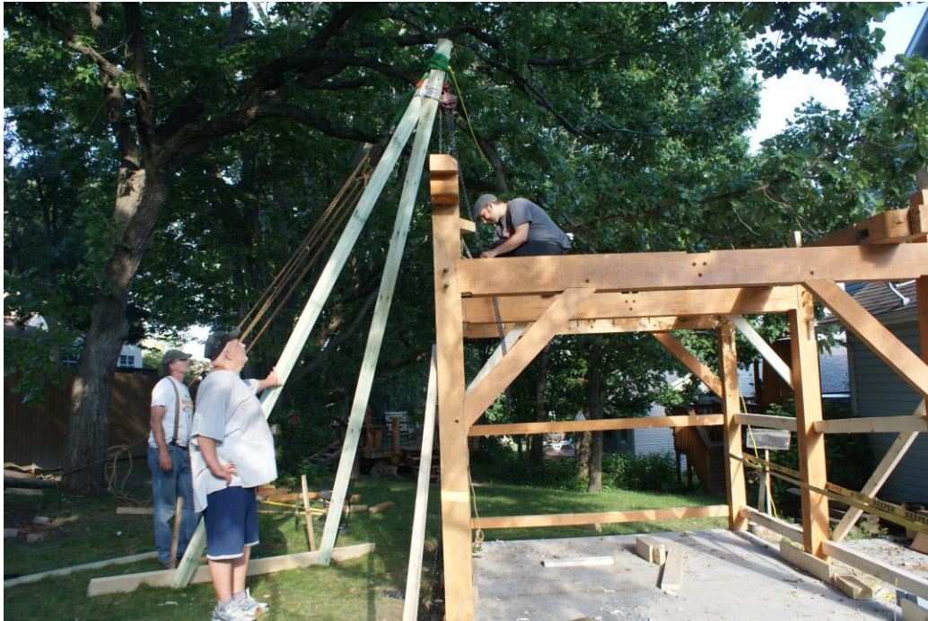
Installing the Plate
