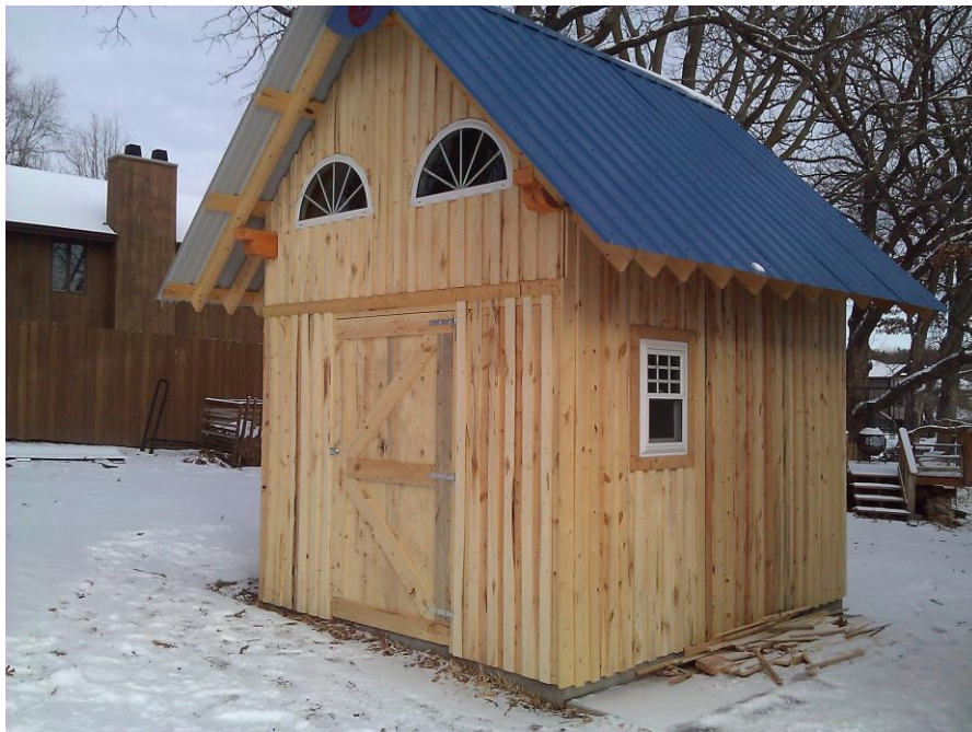
Workshop/Shed Constructed from 6" x 6" Aspen
