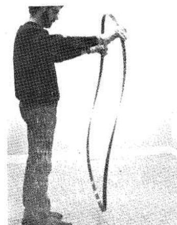
FIGURE B-11. BLADE INVERTING STEP #4.
